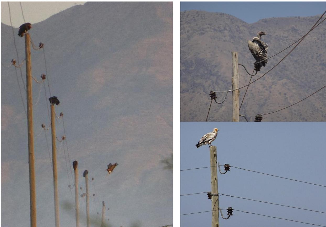
**Fig. 4.** Photos showing one of the surveyed low-voltage power lines next to the local and the export abattoirs, with vultures perched on almost every single pylon. Although this pylon type is less dangerous than the metal crossbar type, vultures get electrocuted when they spread their wings during landing and take-off (photos: V. Arkumarev & S. Oppel).
